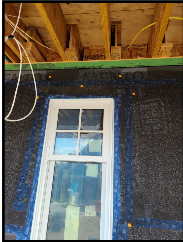
No air barrier between cantilever and conditioned space
