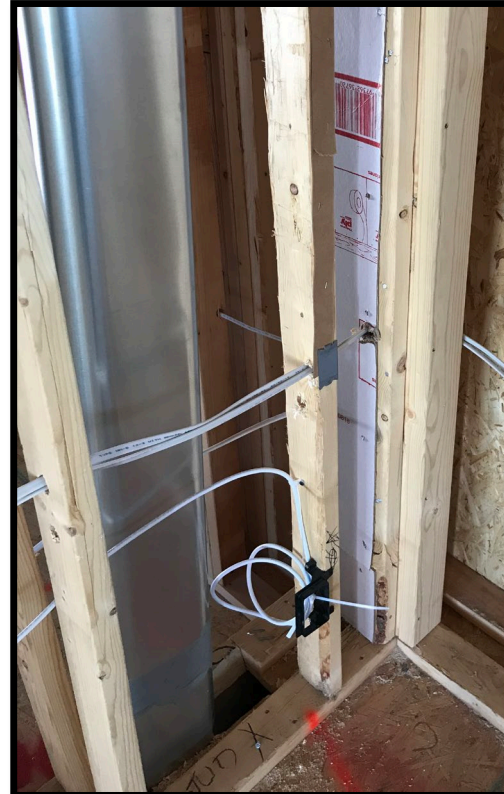
Air Barrier Separating HVAC Chase from Exterior Wall
