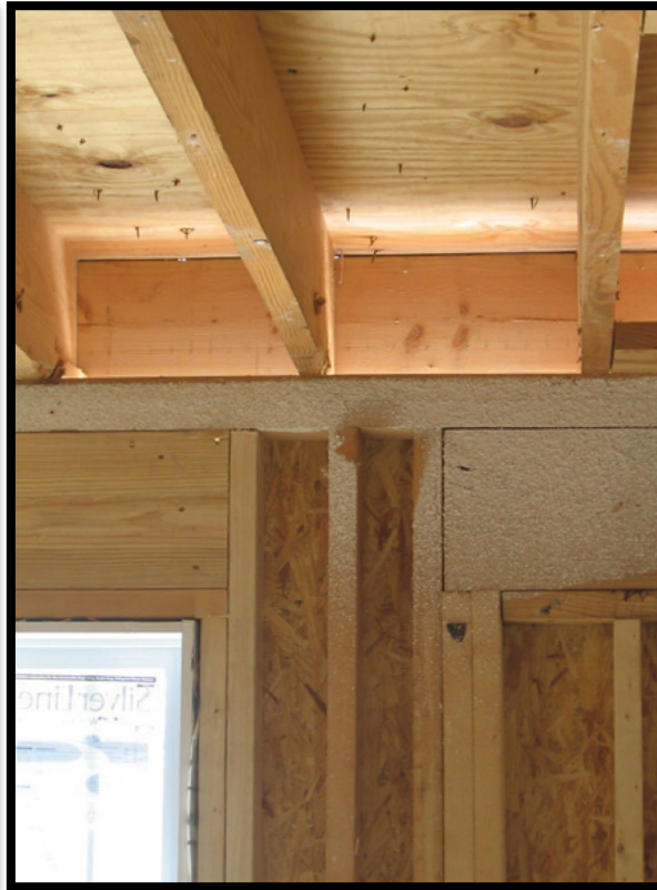
No air barrier between cantilever and conditioned space
