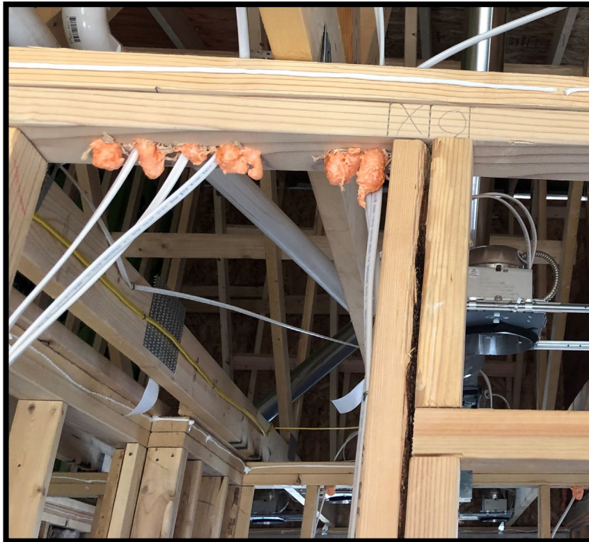
Electrical Penetrations Sealed
