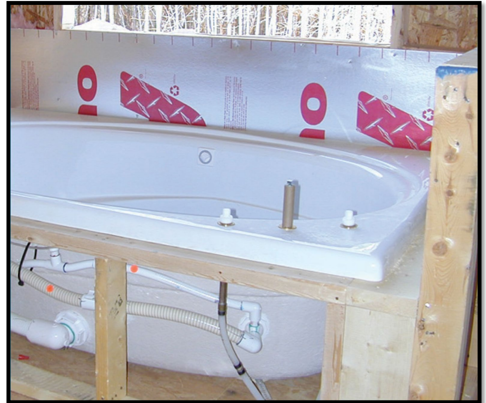
Air barrier in place prior to tub install
