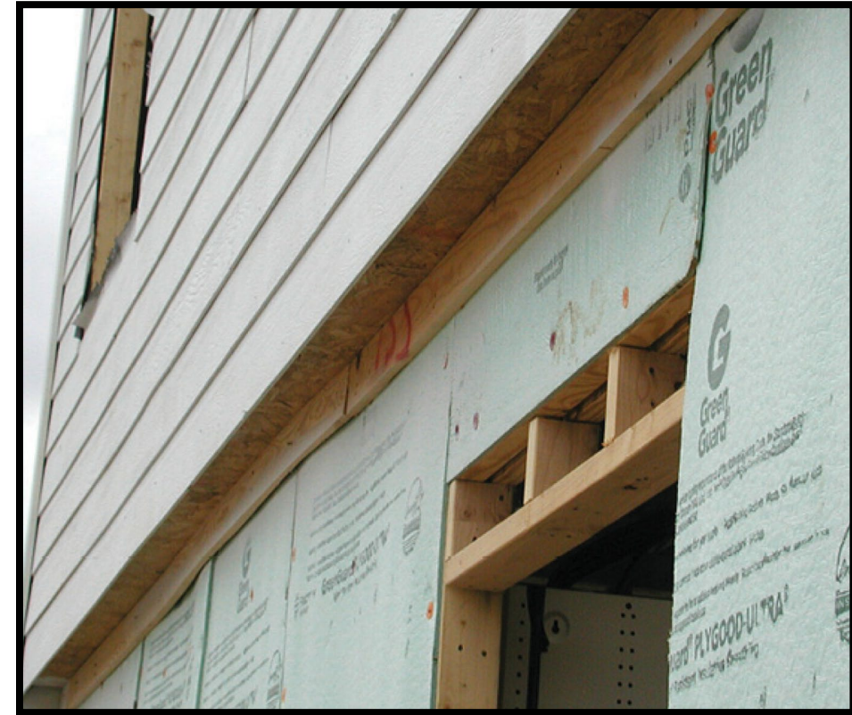
Cantilever properly blocked and sealed
