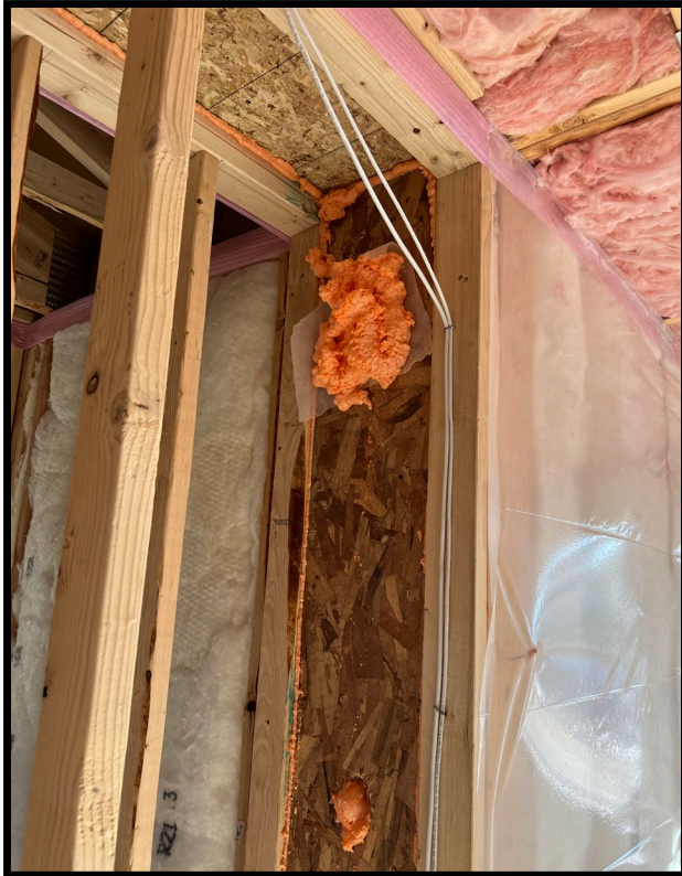
Utility Chase at Exterior Wall
